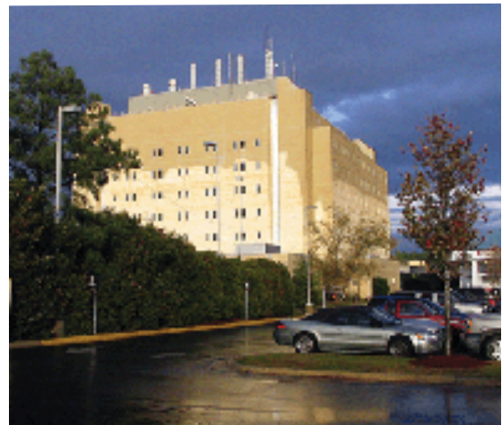
Figure 1: WDR distribution on a building.
